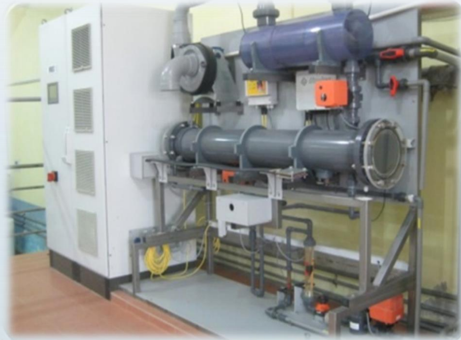
Electro-chlorination System at Salim Water Treatment Plant , Sibü
